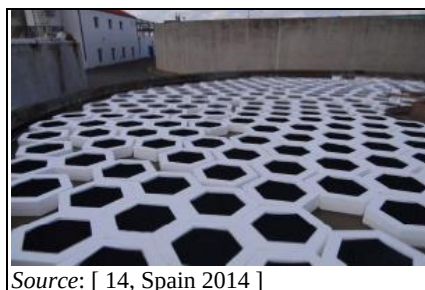
Figure 4.78: Geometrical plastic tiles in a slurry tank
